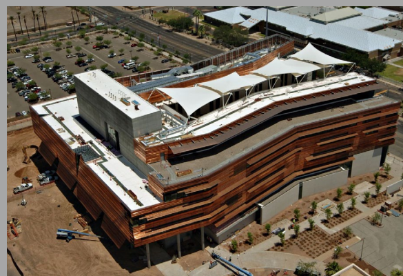
Under Construction - Health Science Education Building
